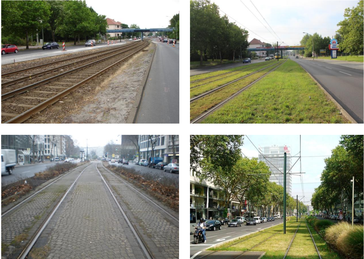
Fig. 9: Tracks before and after greening in Berlin (top; photos Dreger, BVG and Schreiter, IASP) and Düsseldorf (bottom; photos Ahrens, Rheinbahn AG)
