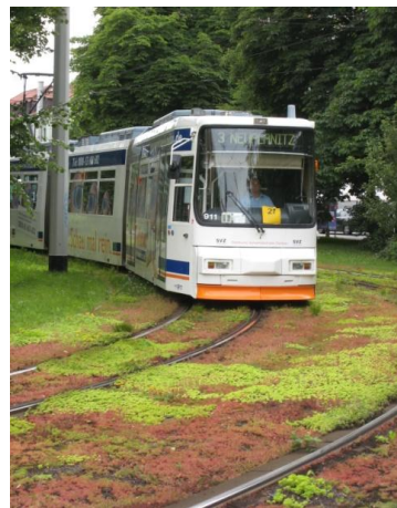
Fig. 7: Vegetation system up to the top of the rail (photo Kappis, IASP)
